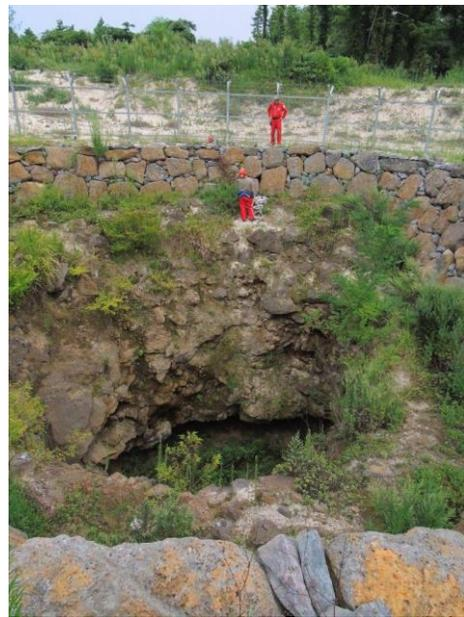
**Figure 19:** Newly dug and secured Opening 3 of Socheon Cave. Note fence and retaining wall around perimeter. At the bottom cave opening leading into newly opened section.
